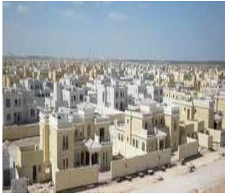
Project: Al Falah Villas - Abudhabi Consultant: Khatib & Alami MEP Contractor: ALEC/EL Mech.JV
