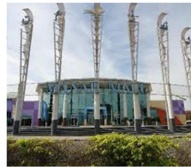
Project: Manar Mall-RAK Consultant: Manar Development Main Contractor: Manar Development MEP Contractor: ETA MNE - DUBAI
