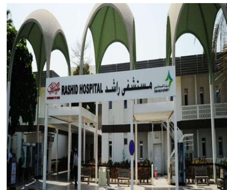
Project: Doh&Ms Rashid Hospital-Dubai Consultant: AL BUR Engineering Main Contractor: Al Habbai Contracting Co MEP Contractor: ETA M&E-Dubai
