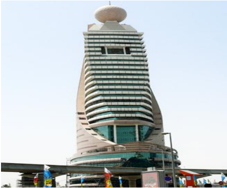
Project: Etisalat Telecom- Dubai Consultant: Dhankland Main Contractor: Arabin Con. MEP Contractor: Mapco
