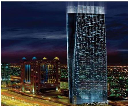
Project: Sama Tower – Dubai Consultant: WS Atkins & Partners MEP Contractor: ETA MNE – Dubai
