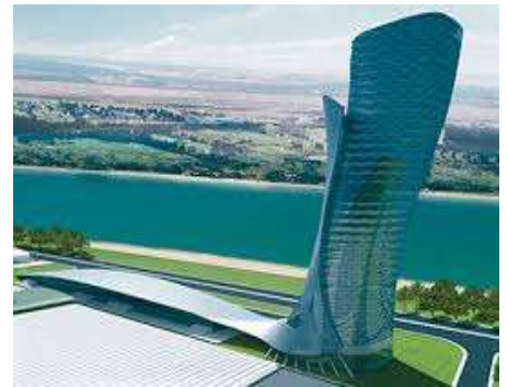
Project:Abudhabi National Exhibition Centre Consultant: RMJM Main Contractor: Al Habthoor MEP Contractor: ETA M&E – Abudhabi
