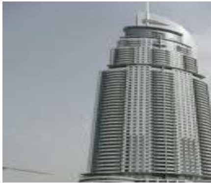
Project: Burj Dubai Lake Hotel-Dubai MEP Contractor: IEMSC
