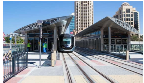
Project: Dubai Tram–DXB Consultant: Systra Main Contractor: BESIX MEP Contractor: ETA & Al Futtaim
