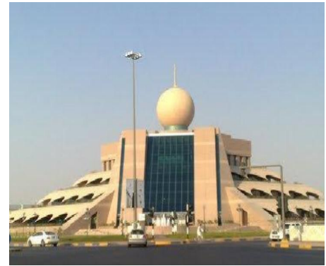
Project: Etisalat Telecom – Al Ain Main Contractor: Arab Tech MEP Contractor: ETA MNE
