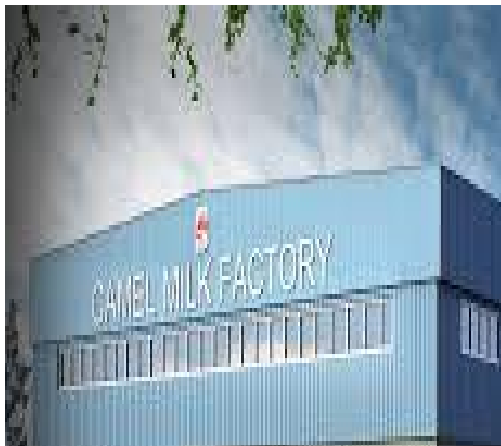
Project: Camel Milk Factory-Al Ain MEP Contractor:Jasaf Building Contracting
