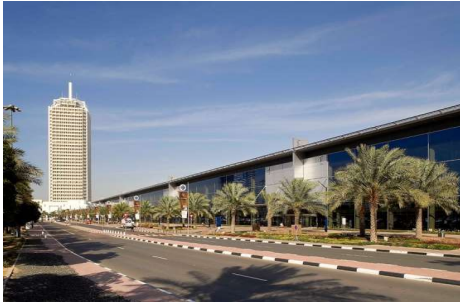
Project: Conventional Centre –DXB Consultant: RMJM Main Contractor: Khansaheb MEP Contractor:ETA MNE - Dubai
