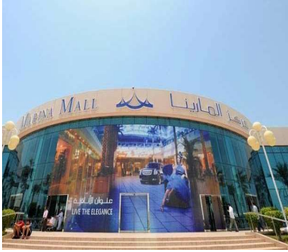
Project: Marina Mall–Abudhabi Consultant: Mein Hardc Singapore PV Main Contractor: ALEC Contracting LLC MEP Contractor:ETA MNE –Abudhabi
