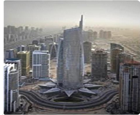
Project: Al Mas Tower– Dubai Consultant: WS Atkins & Partners Main Contractor: Arabian Construction Company MEP Contractor: ETA MNE – Dubai
