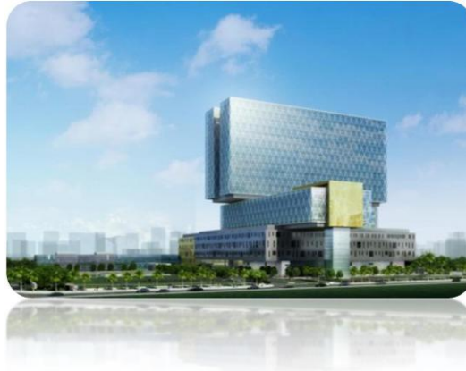
Project: Cleveland Clinic–Abudhabi Consultant: KEO Consultant Main Contractor: BESIX & SAMSUNG JV MEP Contractor: ETA M&E -Abudhabi
