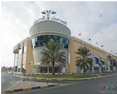
Project:Al Ain Mall– Al Ain Consultant: Khatib & Alami Main Contractor: Al Farah Group MEP Contractor: Al Sabah Electro Mech.
