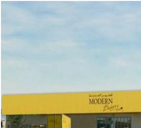
Project: Modern Bakery - Dubai MEP Contractor : IEMSC
