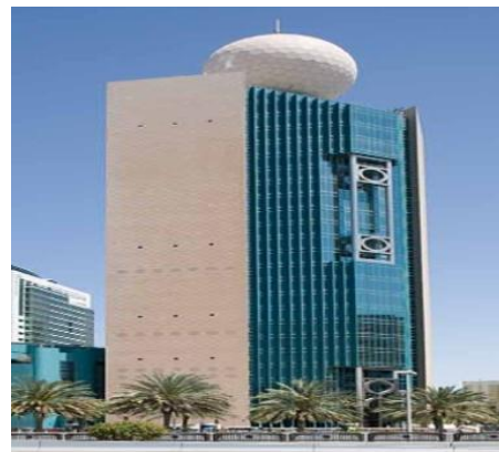
Project: Etisalat Telecom - Abu Dhabi
