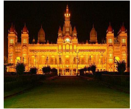
Project: Al Rawdha Palace –Al Ain Consultant: WS Atkins Main Contractor: BESIX & Arabtech MEP Contractor: Omega Engineering
