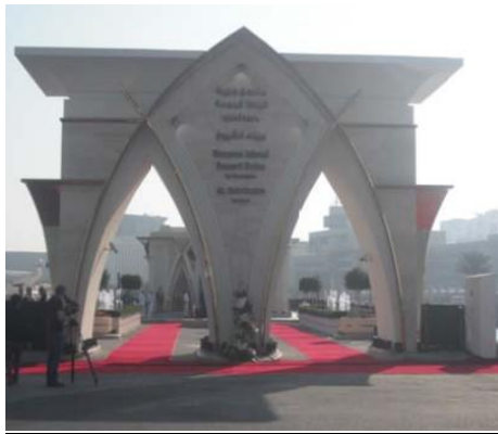
Project: Banana Island Resort Consultant:Engineering Consultant Group MEP Contractor : Radiant Engineering Enterprises
