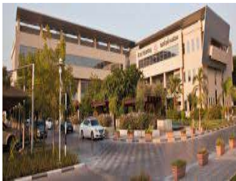
Project: Ras Al Kaimah Hospital-RAK Consultant: Ian Banham & Associates Main Contractor: ASCON, Dubai MEP Contractor: ETA M&E-Dubai
