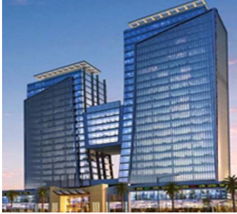
Project: Shemoukh Twin Tower Consultant: SEG MEP Contractor: Arabian MEP Contracting.
