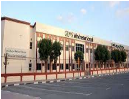
Project: GEMS School – Dubai MEP Contractor:Chicaco Contracting.
