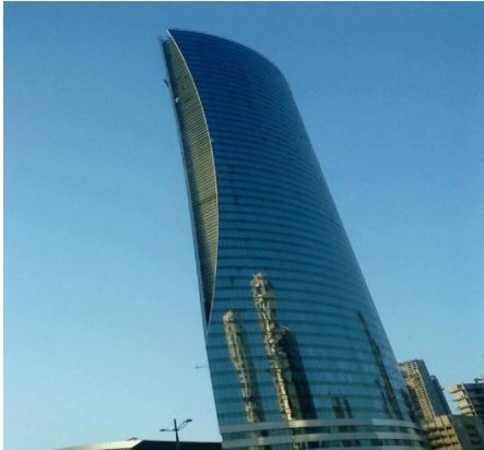
Project : Qatar Navigation Tower Consultant: MZ & Partners MEP Contractor: ETA MNE
