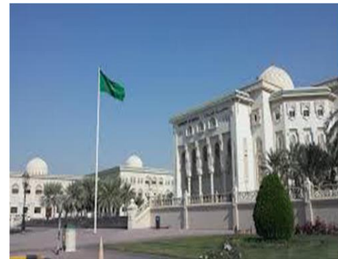
Project: Etisalat College Of Engineering -SHJ MEP Contractor: GECO Mech & Electrical.
