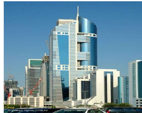
Project: HHHR Tower - Dubai Consultant: Al Hashmi MEP Contractor: ETA MNE – Dubai
