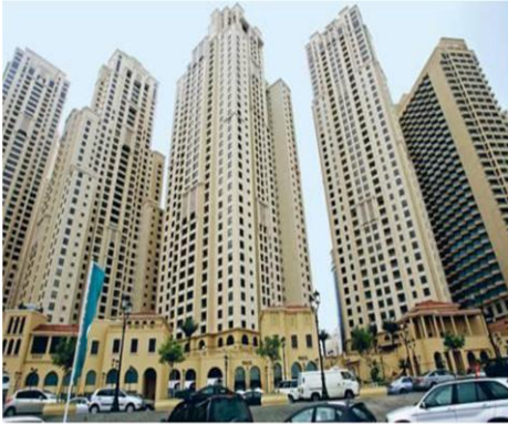
Project: Jumeirah Beach Res. Consultant: WS Atkins & Partners Main Contractor: Al Ahmadiyah Contracting. MEP Contractor: ETA MNE – Dubai
