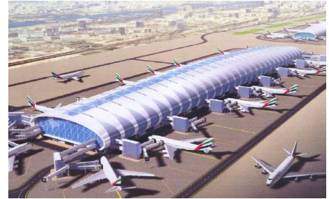
Project: Dubai Int.Airport C3-DXB Consultant: DAR Al Handasah Main Contractor: ALEC MEP Contractor:ETA MNE –Dubai
