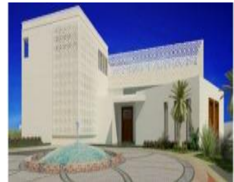
Project: Ibrahim Mahmoud Villa Consultant: ERGA Qatar MEP Contractor: Radiant Engineering
