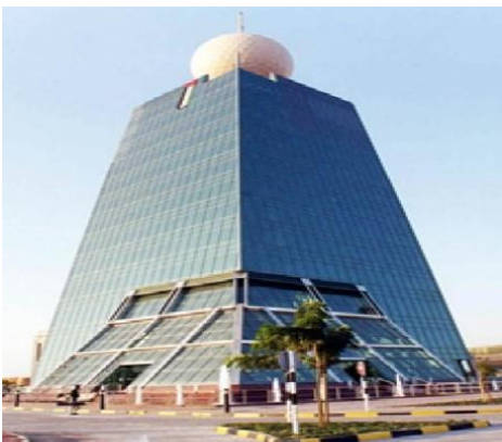
Project: Etisalat Telecom – Ajman MEP Contractor: Energo Project
