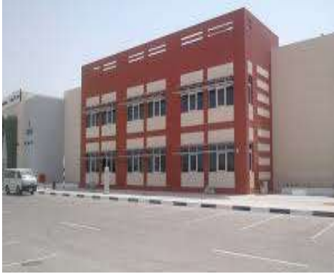
Project: Abudhabi Future School –Baniyas Consultant:Dewan Consultant Main Contractor: AMANA Contracting MEP Contractor: ETA MNE – Abudhabi
