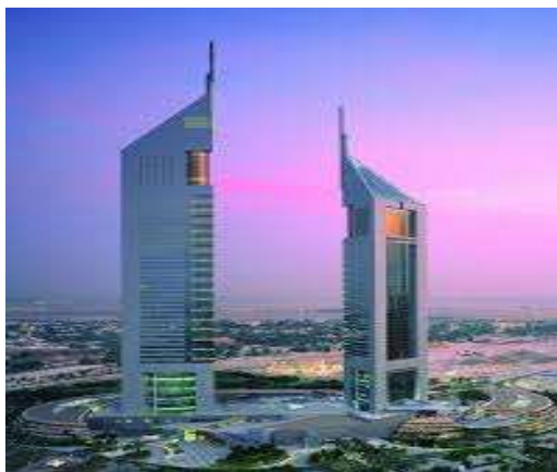
Project: Emirates Towers-Dubai MEP Contractor: ETA MNE – Dubai
