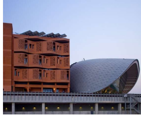
Project: Mazdar Institute Of Science -Abudhabi MEP Contractor: STS – Abudhabi
