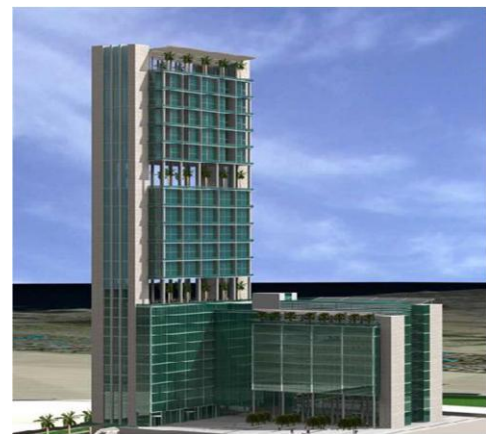
Project: Liberty House-Dubai MEP Contractor: ETA MNE – Dubai
