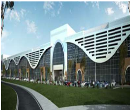
Project: Barwa Commercial Avenue-Ph-I & II Consultant : AECOM Middle East MEPContractor : ETA M&E
