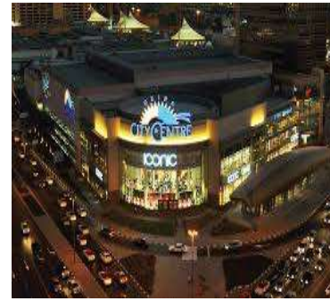
Project: Deira city centre -Dubai MEP Contractor:ETA MNE –Dubai
